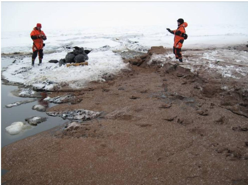
Figure 5.16: After collection of residue the area was treated with bark to immobilise any small quantities of remaining residue. The waste bags with collected residue and adsorption pads can also be seen in the photo.
