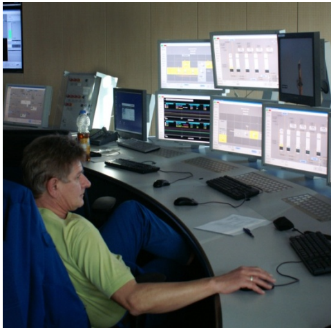
Control room operator
