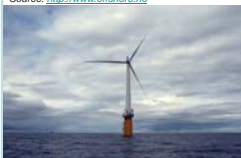
Figure: Hywind turbine outside Karmøy, Norway. Source: http://www.offshore.no
