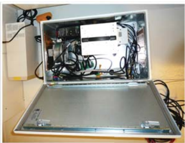
Figure 2 EMC box installed in the transformer platform at Gunfleet Sands Offshore Wind Farm.
