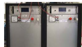
60 kVA AC/DC converter units with inhouse developed FPGA based control system.
