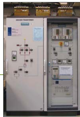
Transformer substation, model with busbar and protection relays typical for 66kV/22kV substation.
