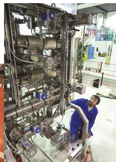
Torrefaction unit (Trondheim)
