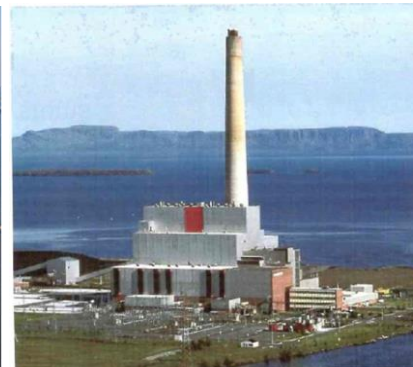
2013 & 2014 Thunder Bay, Canada 312 MW power station Dedicated 100 % capacity
