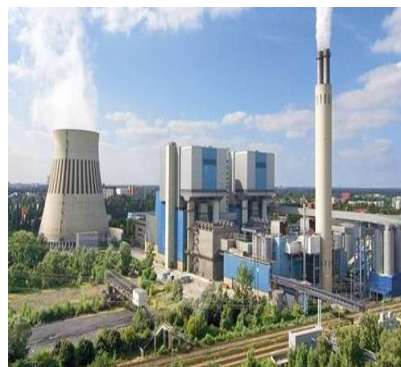
2011 Reuter West, Berlin Germany 2 * 300 MW power station Co-firing 20% to 50%
