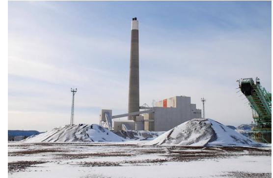
Thunder Bay GS – world first full conversion to Advanced Wood Pellets
