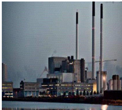
2012 Amager, Denmark 250 MW CHP
