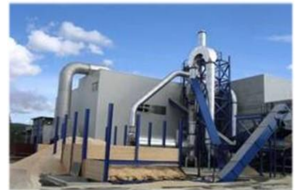
Grasmo Steam Explosion Pellet Plant - built in 2003
