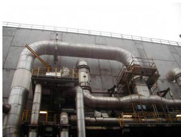
Figure 6: New prefabricated mixer element (top) and installation on site (bottom).
